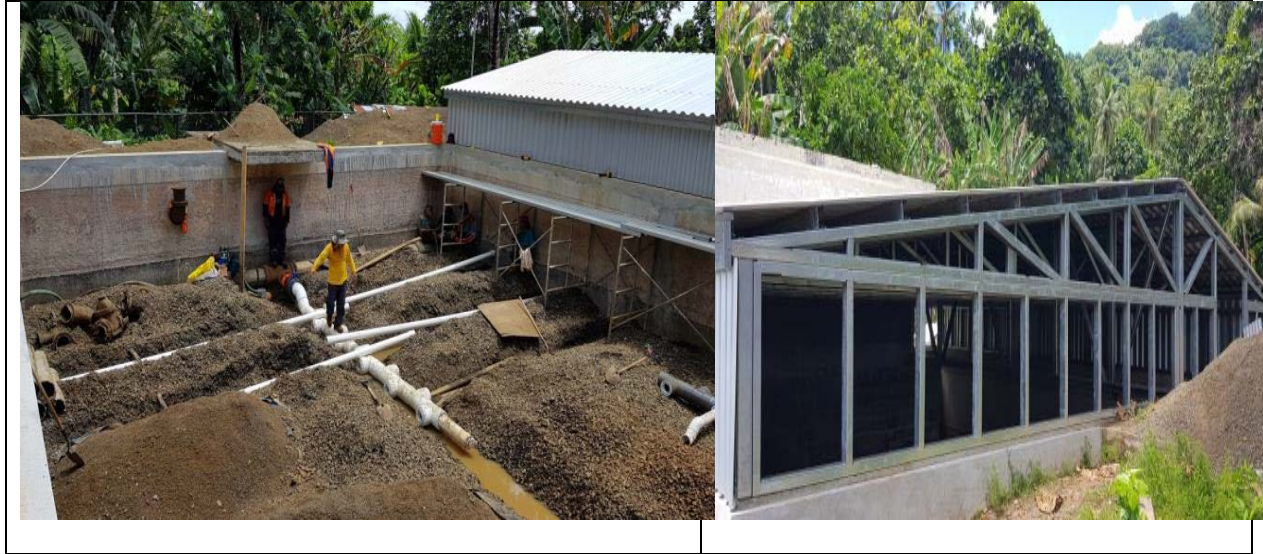
Filter Underdrain system being installed
