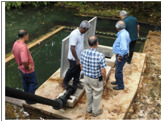
Inspecting the Intake Structure
