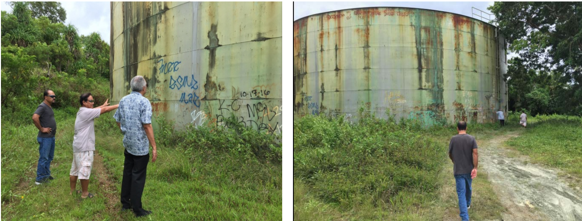
Site Inspection at Tank No. 2
