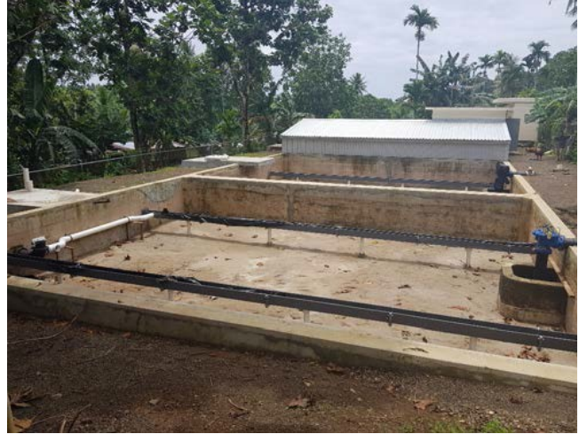
Pic 2: Rehabilitated WTP (Civil Works Completed Aug 2018)
