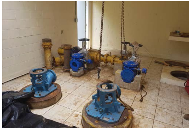
Pic 5: Pump House with new pumps (under construction)
