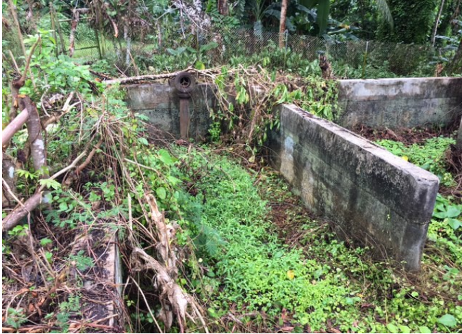
Pic 1: Abandoned Water Treatment Plant (Jan 2018)
