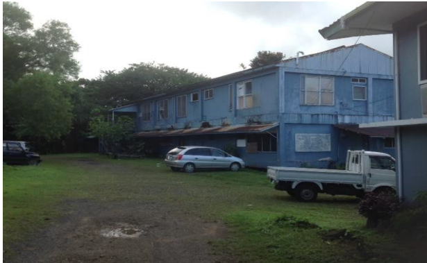
COM Demolition Site Before
