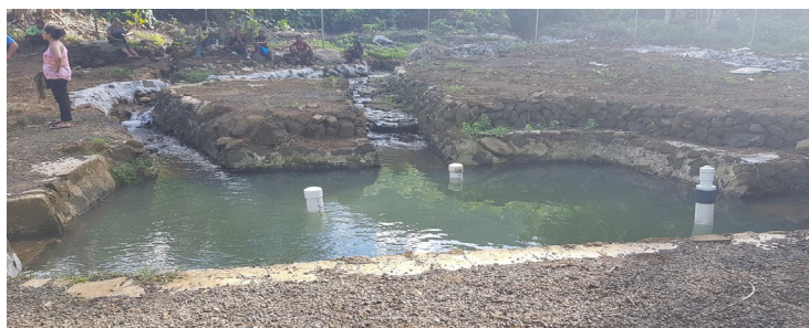
Rehabilitated Fansinifo Intake
