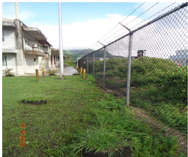
along Front of Dock Warehouse
