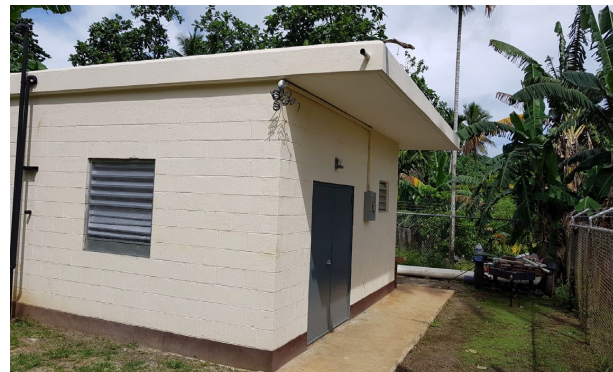
Generator building Nov 2018
