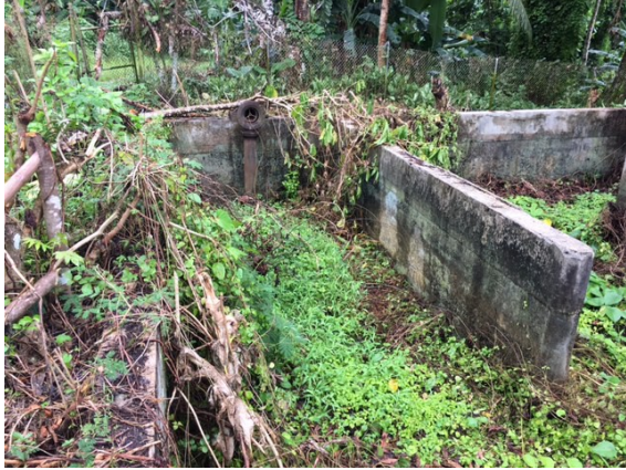
Abandoned Water Treatment Plant (Jan 2018)
