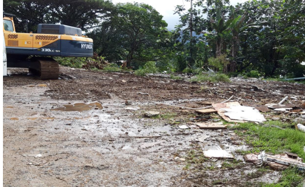
COM Demolition Site After
