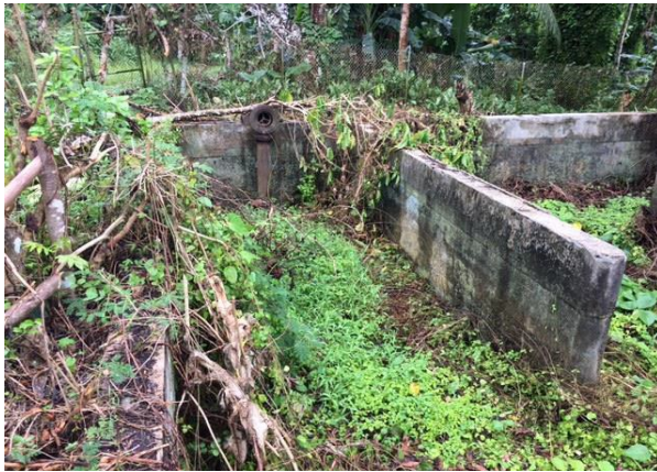
Abandoned Water Treatment Plant (Jan 2018)
