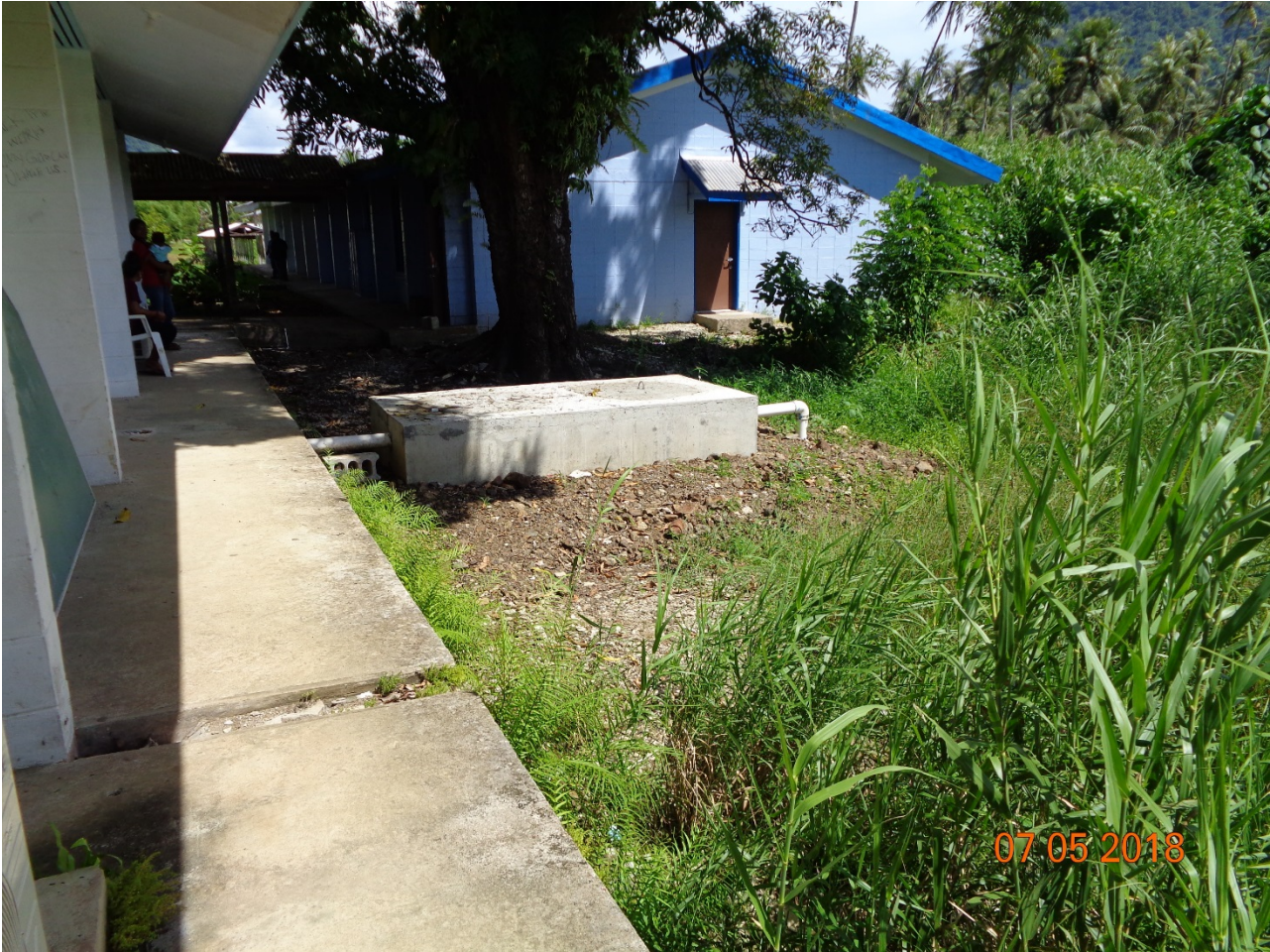
Septic Tank Completed
