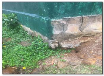
**BLDG 1: FOUNDATION FLEXURAL CRACK**
