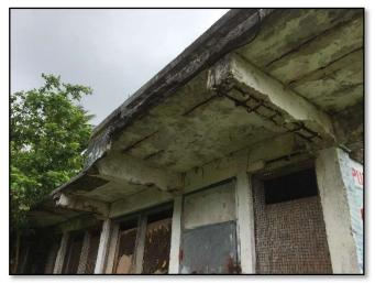
**CONCRETE SPALLING AT BLDG 2**
