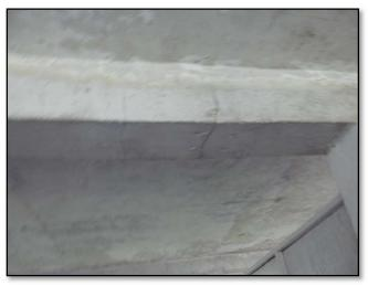
TENSION CRACK ON BEAM AT BLDG 1
