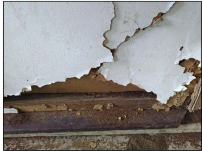
WALL MADE OF THIN FIBER BOARD
