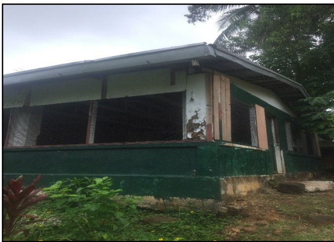
BUILDING 1 SOUTH WEST VIEW
