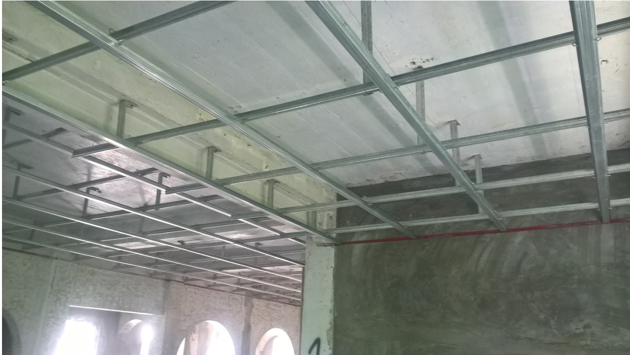
Completed ceiling grid installation at the Main Building
