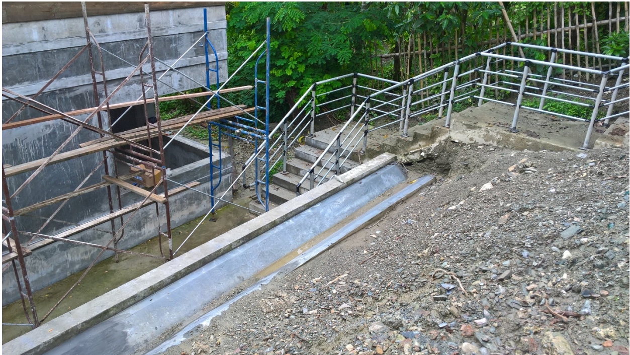
Completed drainage swale and fabricated stair railings
