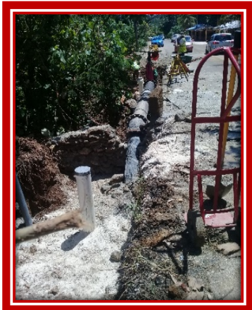
(August 2020 Activities) Storage Tank Site Works & Inlet Pipeline Installation:
