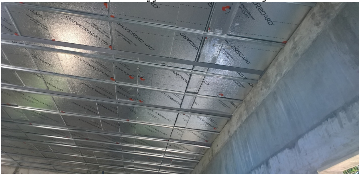
Completely installed ceiling insulation for the Annexes
