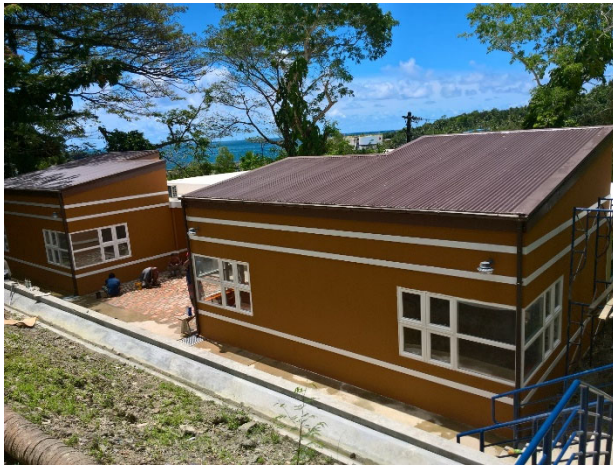
Completed exterior painting works.
