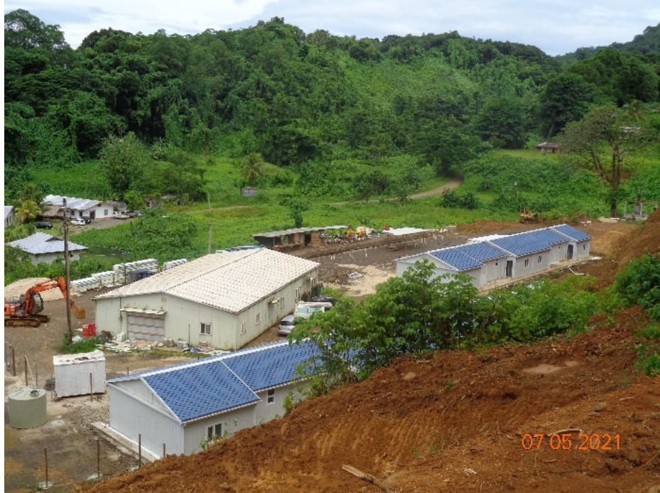
Quarantine Facility in Kosrae – nearing completion
