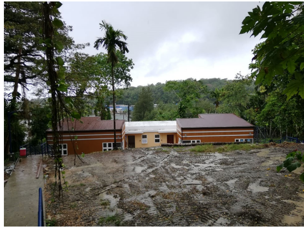
Site upper portion was graded for parking area.
