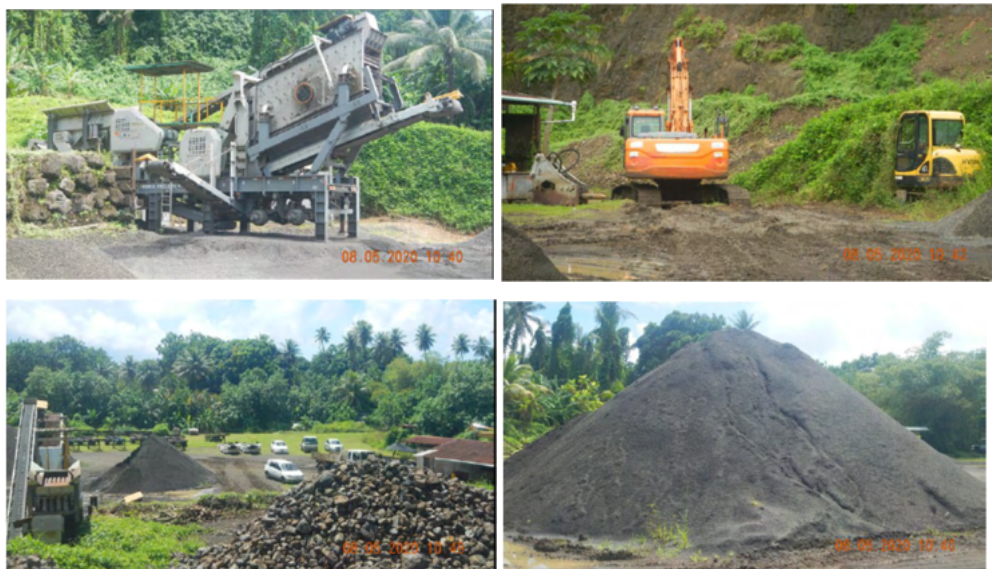
Figure 3-13: Images showing infrastructure at Puk quarry
